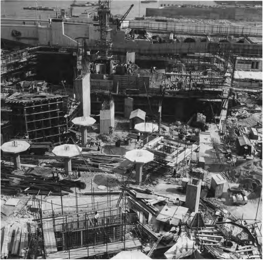
Early stages of construction. Source: Photograph courtesy of Rod Bond
