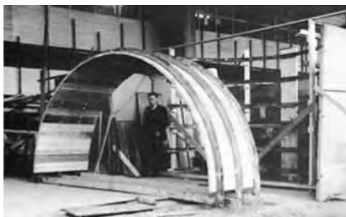
Formwork for spiral staircase. Source: Crown Journal
