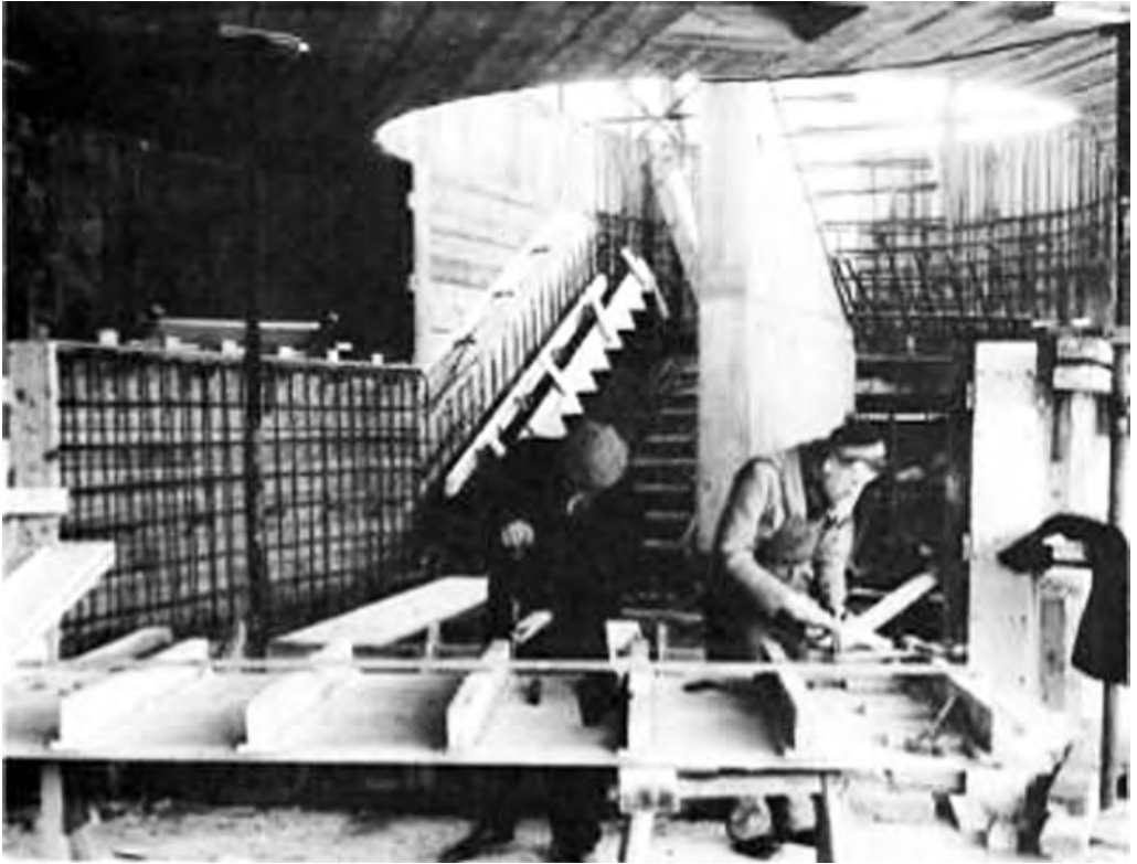
Carpenters working on site on formwork. Source: Crown Journal
