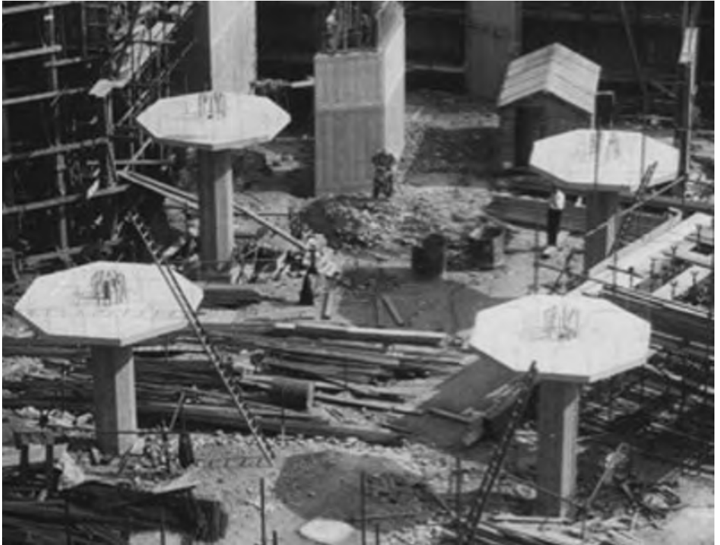
Mushroom columns. Source: Photograph courtesy of Rod Bond
