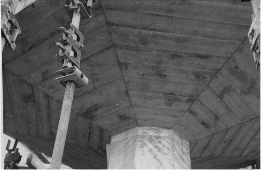
Mushroom column detail. Source: Photograph courtesy of Rod Bond
