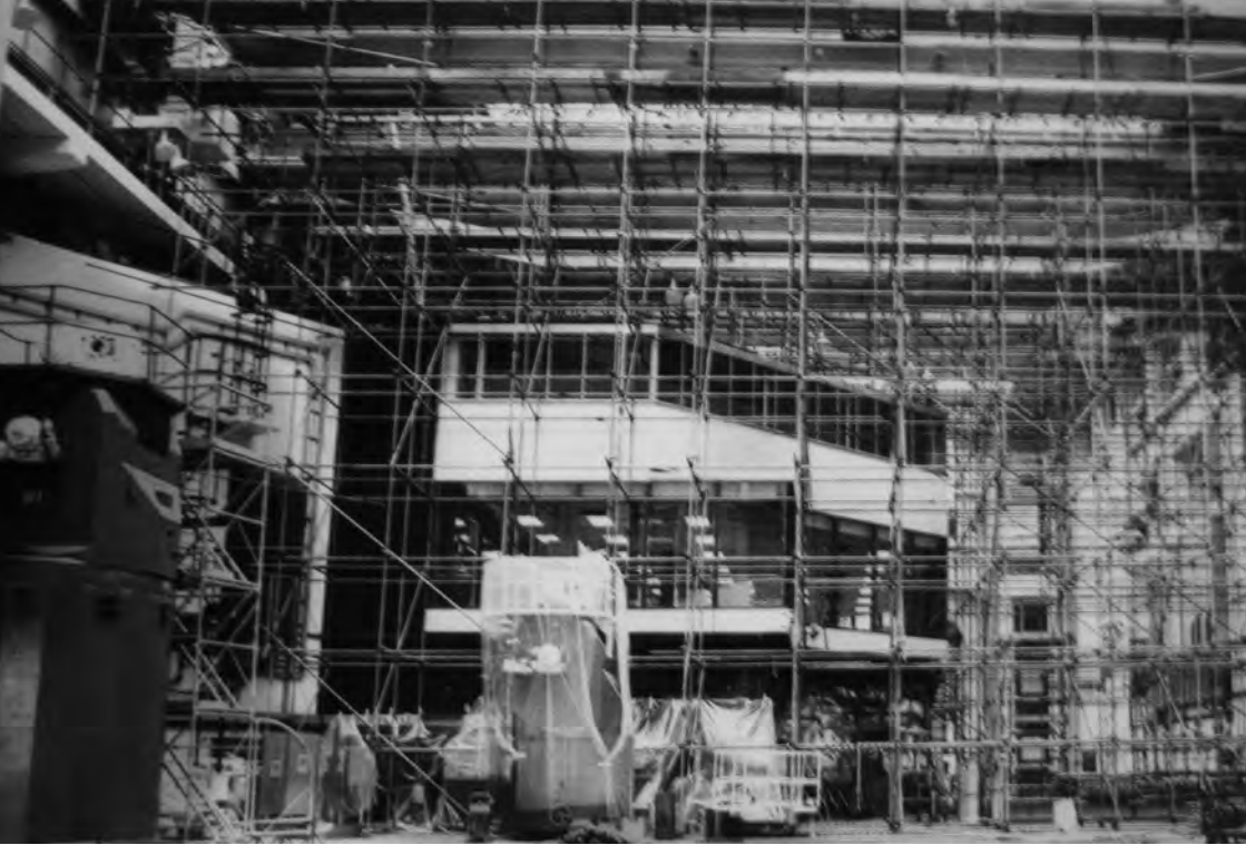
Interior scaffolding. Source: Pat Cable
