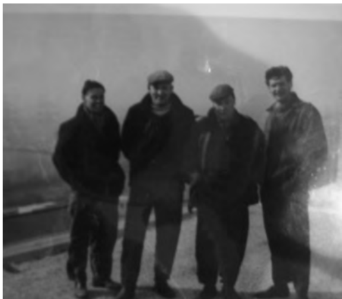
Pat Cable (far right) and a group of workers standing on top of the reactor building. Source: Pat Cable
