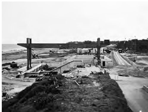
View of cold water pump house under construction. Source: Clive Warneford
