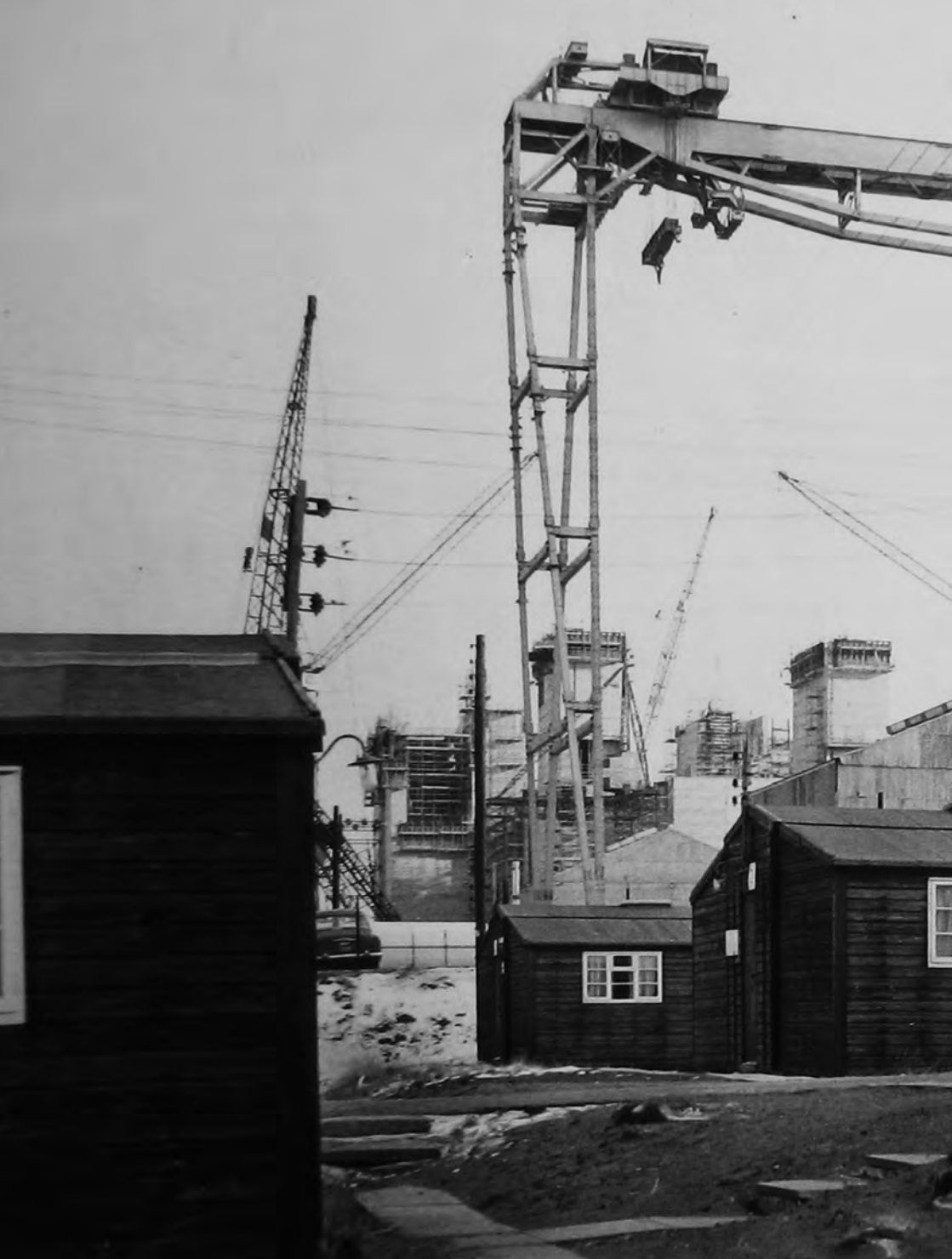
Crane towering over site huts. Source: Charlie Dennis
