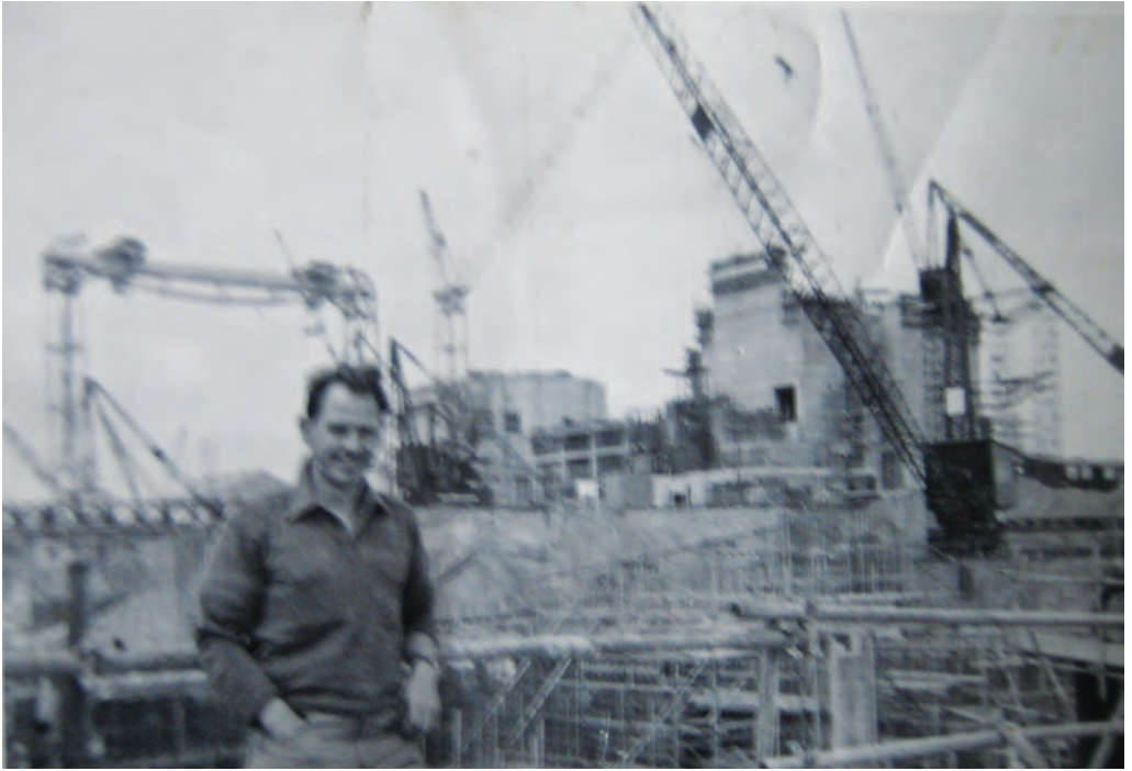
Worker on site. Source: Patrick O’Kane
