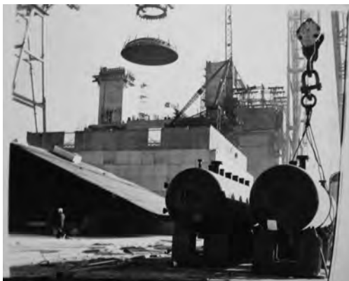
Reactor cap lifted into position. Source: Charlie Dennis
