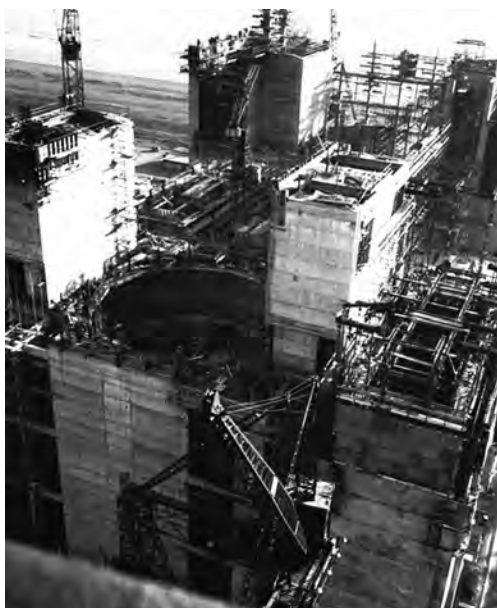
Construction of reactor building c. 1963. Source: Magnox Limited
