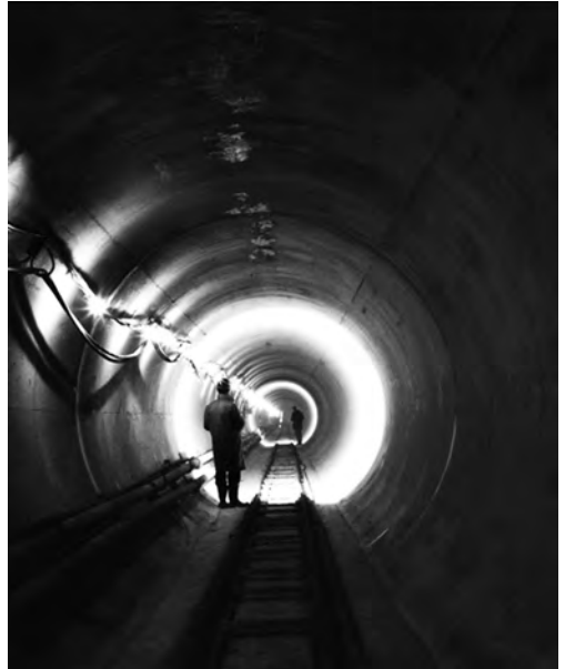
Outfall tunnel during construction phase. Source: Magnox Limited
