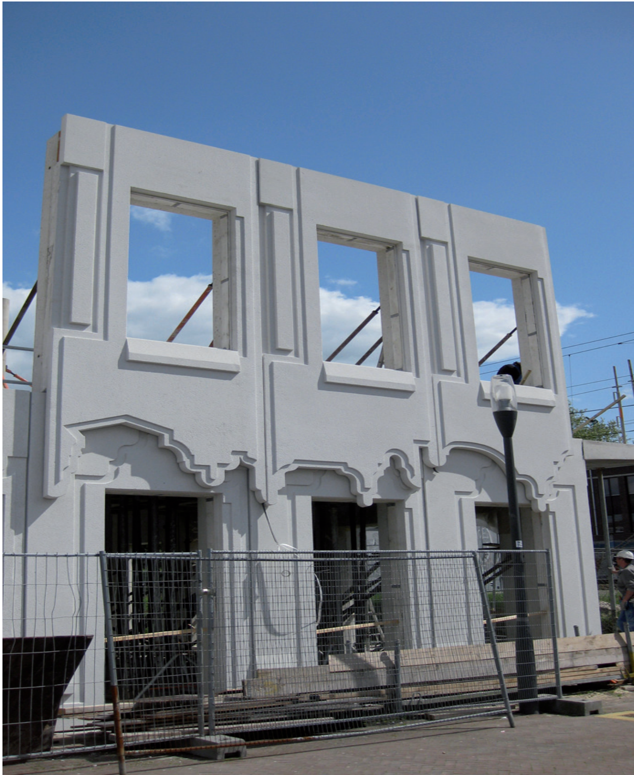
Fig.0 7 Façade panels being erected
