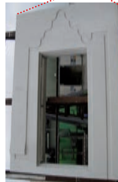
Ground floor panel This needs to be set back to the specified depth, 50mm
