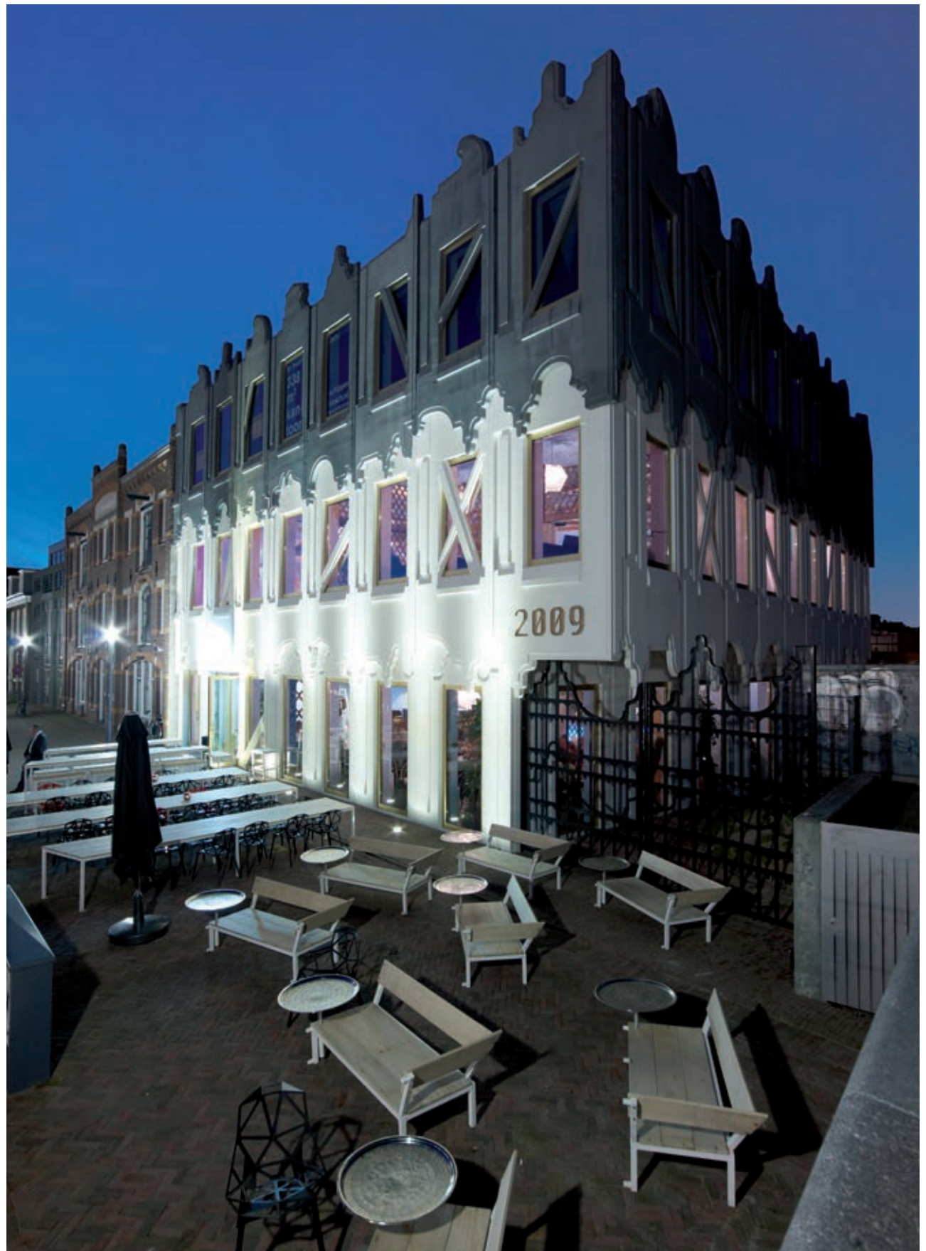
Fig. 10 Corner of building at night
