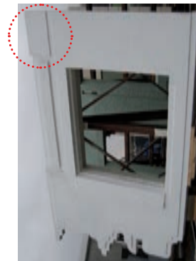
First floor panel This needs to be set back to the specified depth, 50mm
