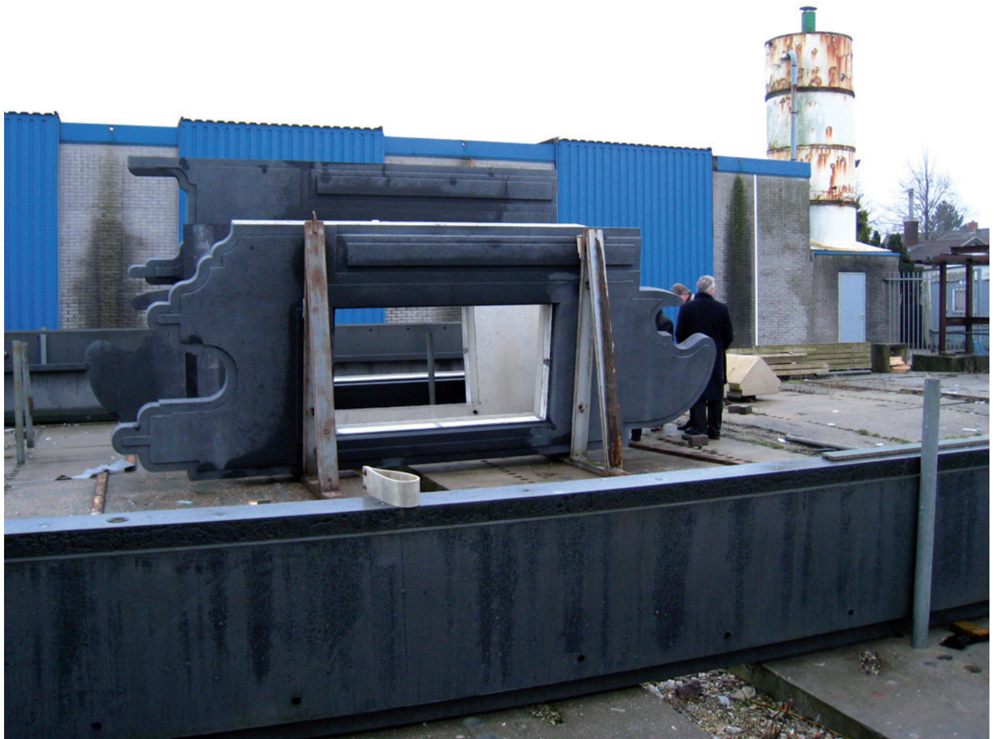
Fig.06 Façade panel in factory
