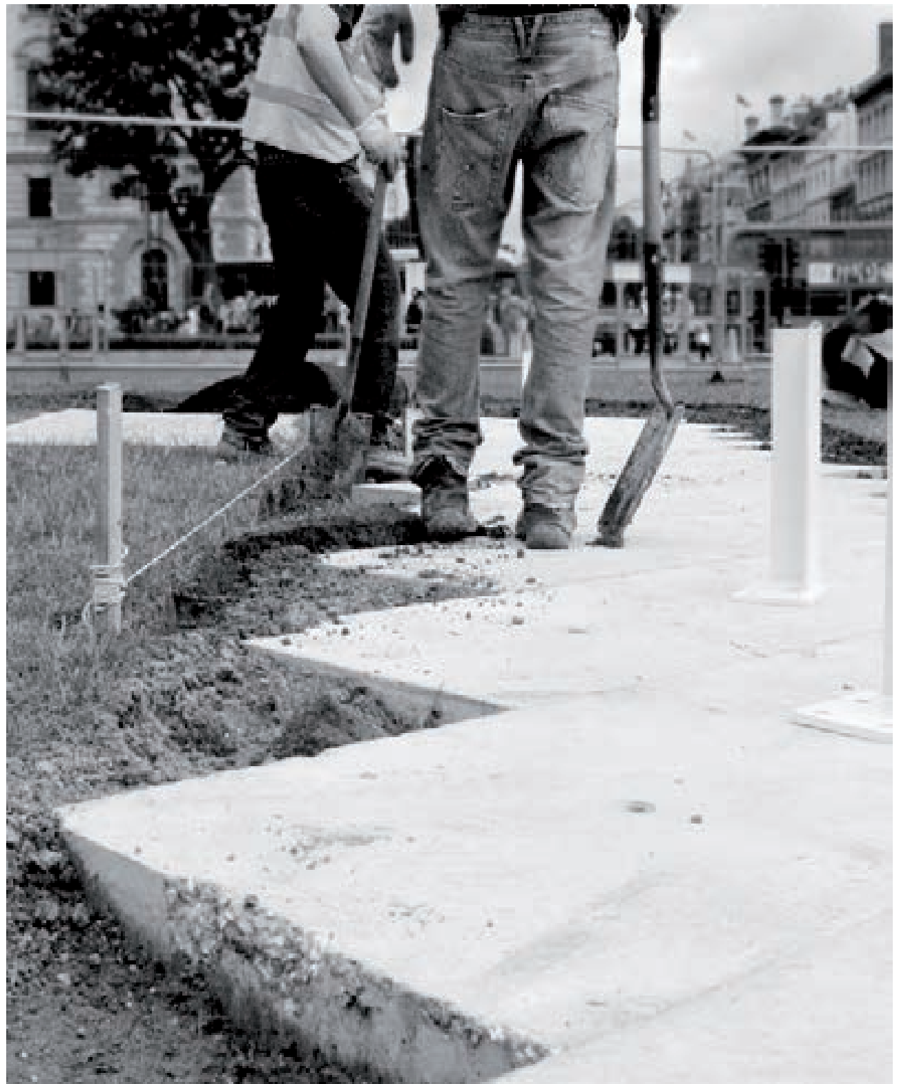
Fig. 28 Precast concrete foundation
