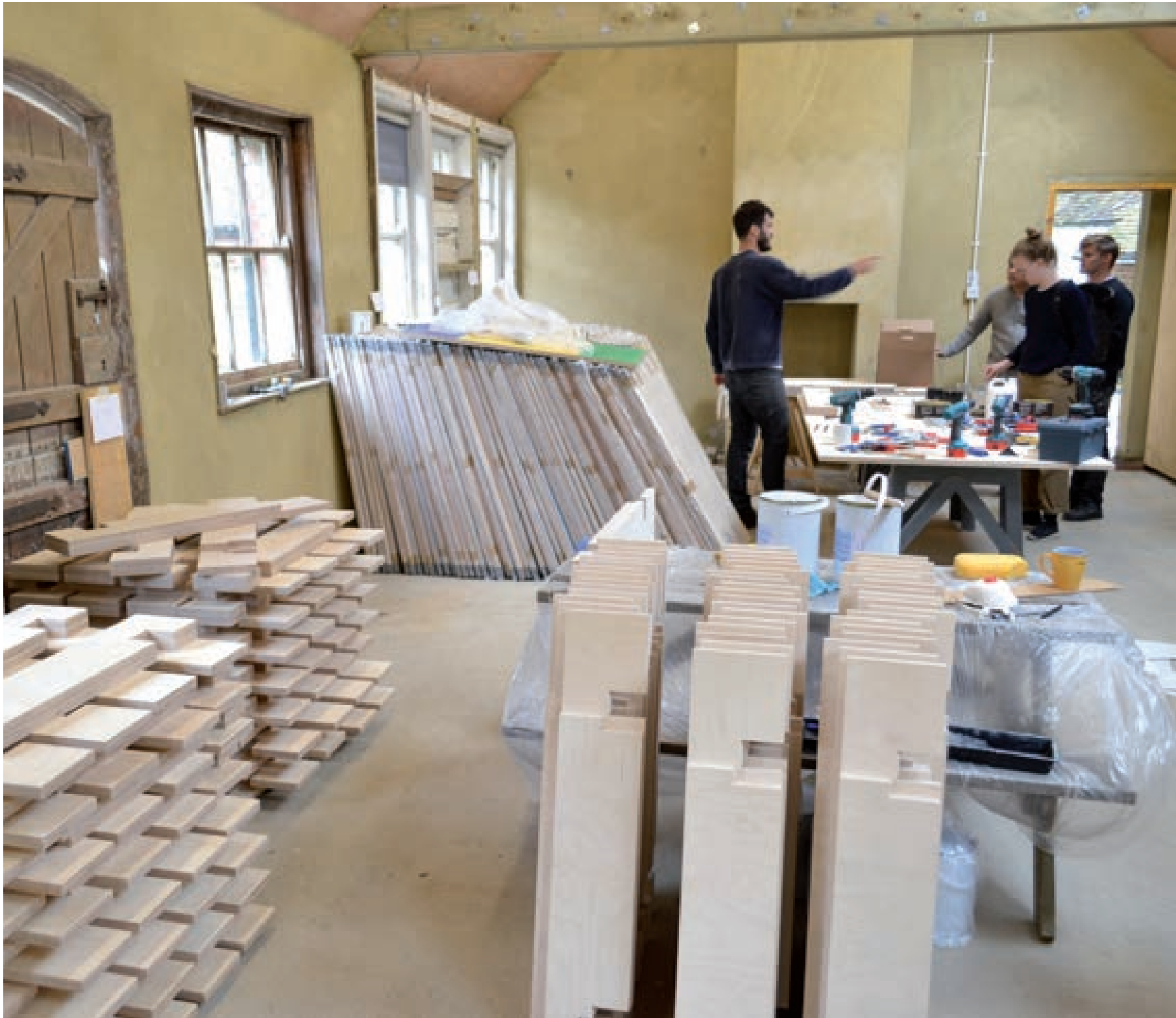
Fig. 18 Fabrication of panels and connections, Grymsdyke Farm, Buckinghamshire
