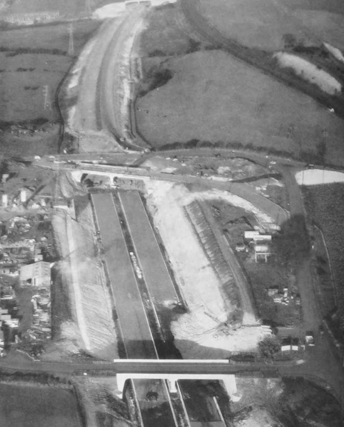
Motorway at Chalton Cross. Source: John Laing archive
