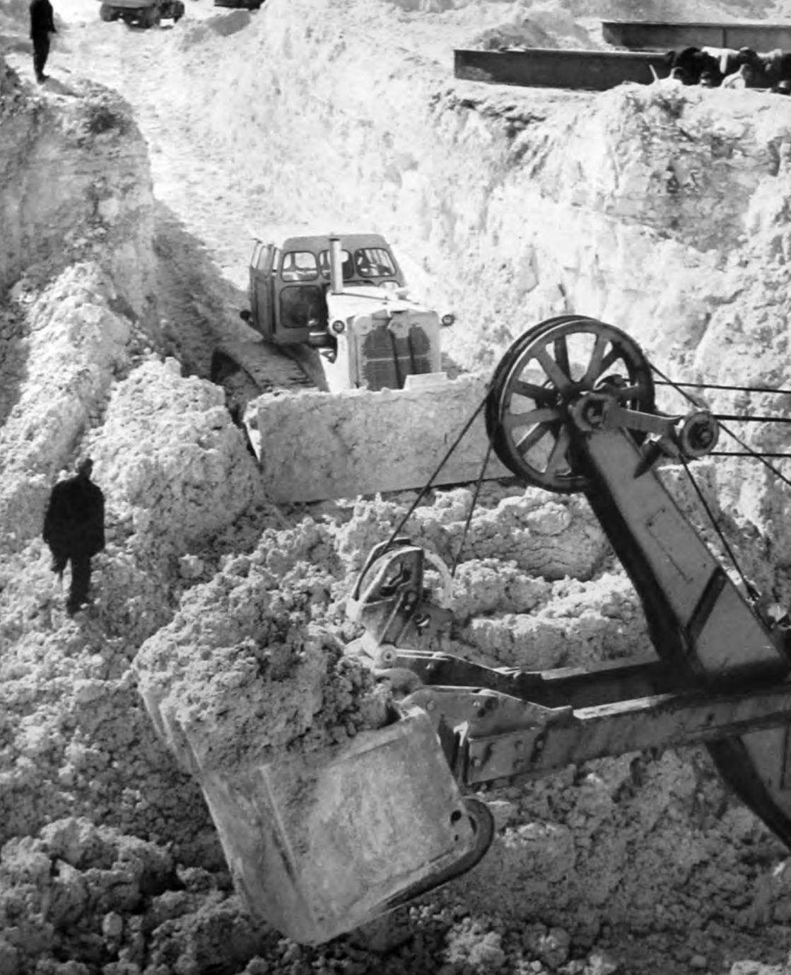
Excavating cutting in chalk near Luton. Source: John Laing archive
