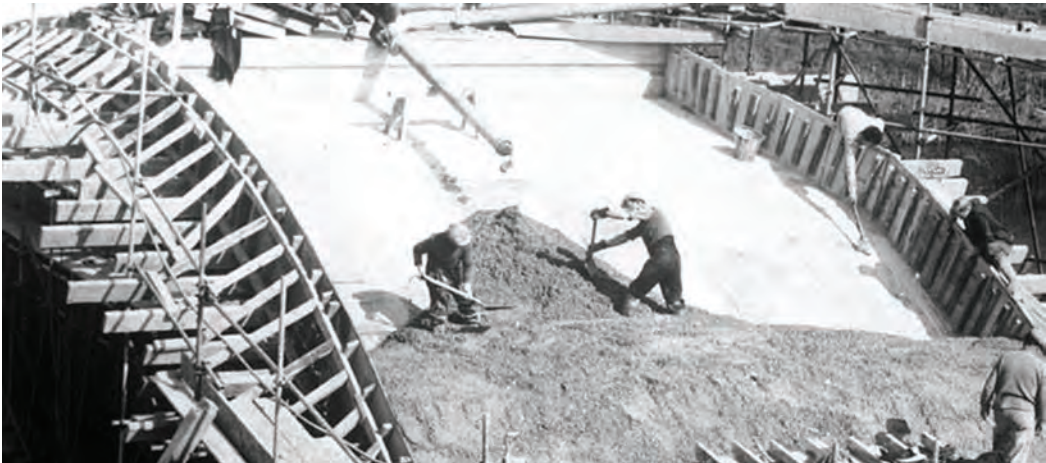
Spreading the concrete at river Ouse viaduct. Source: John Laing archive
