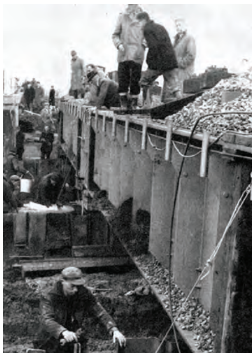
Workers building a railway bridge. Source: John Laing archive
