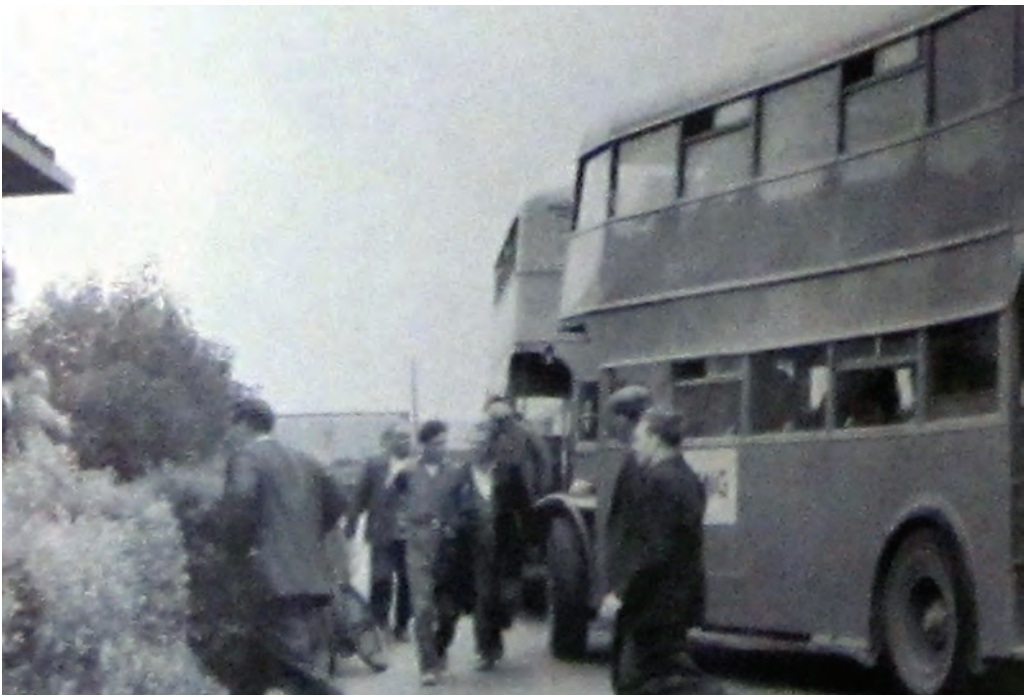
Workers arriving at site on bus. Source: John Laing archive
