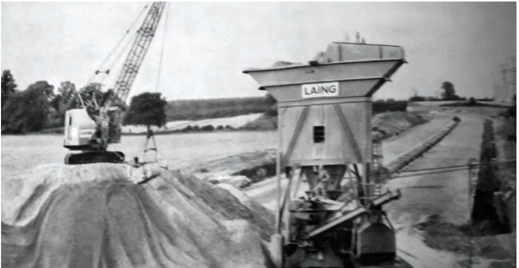
Concrete batching plant. Source: John Laing archive
