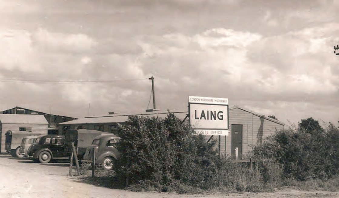
Laing site offices at Hanslope, section C1. Source: Steve Morris
