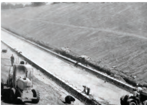
Building the marginal haunches. Source: John Laing archive
