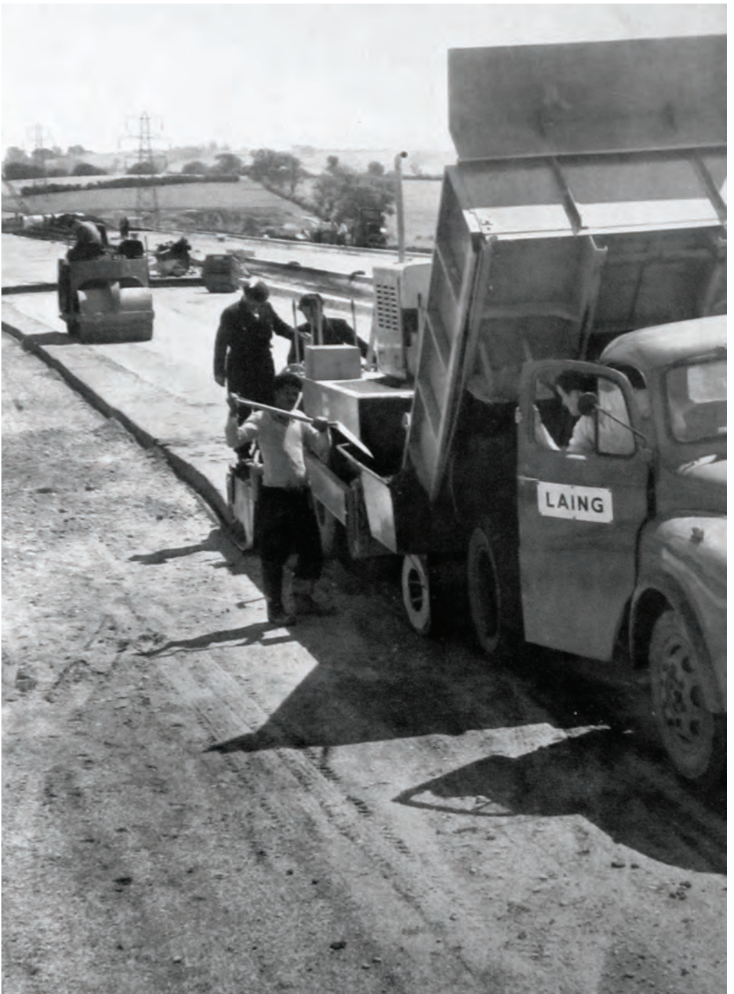
Laying and rolling the lean concrete base. Source: John Laing archive
