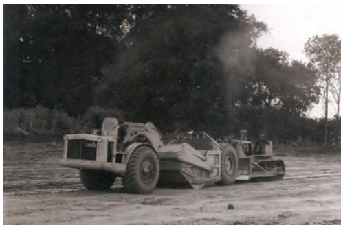
Excavating the M1 . Source: Steve Morris
