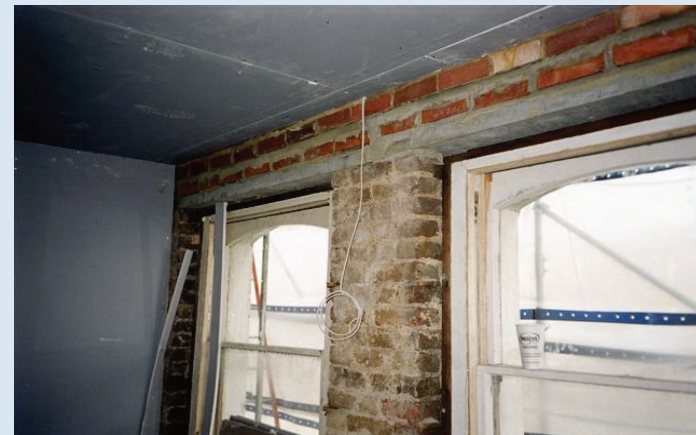
Solid wall insulation and secondary glazing being installed at the property
