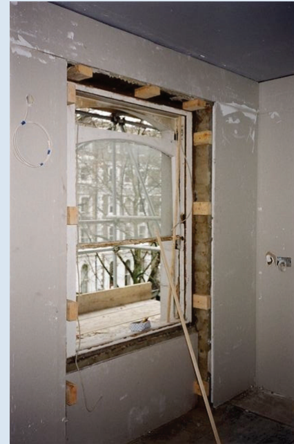
Solid wall insulation and secondary glazing being installed at the property
