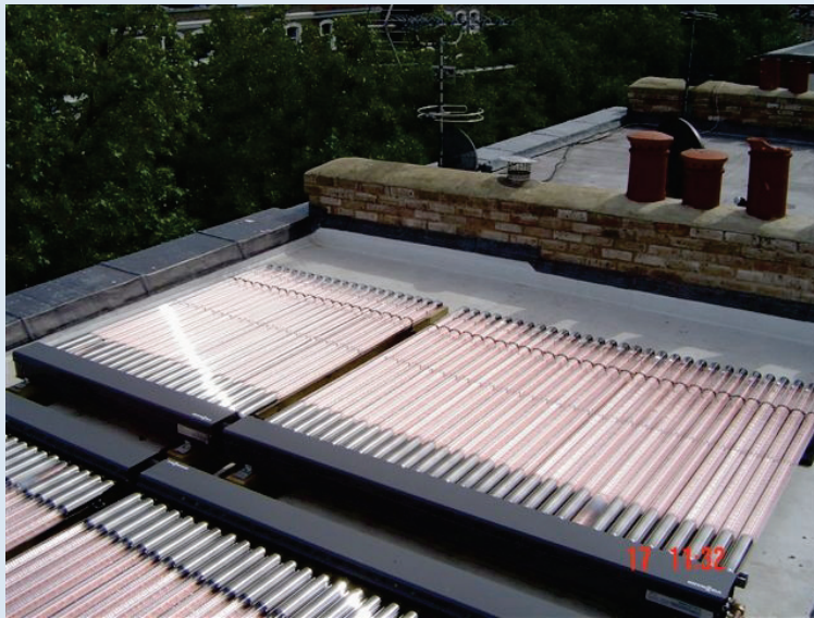
Installed Solar Thermal Panels on the roof
