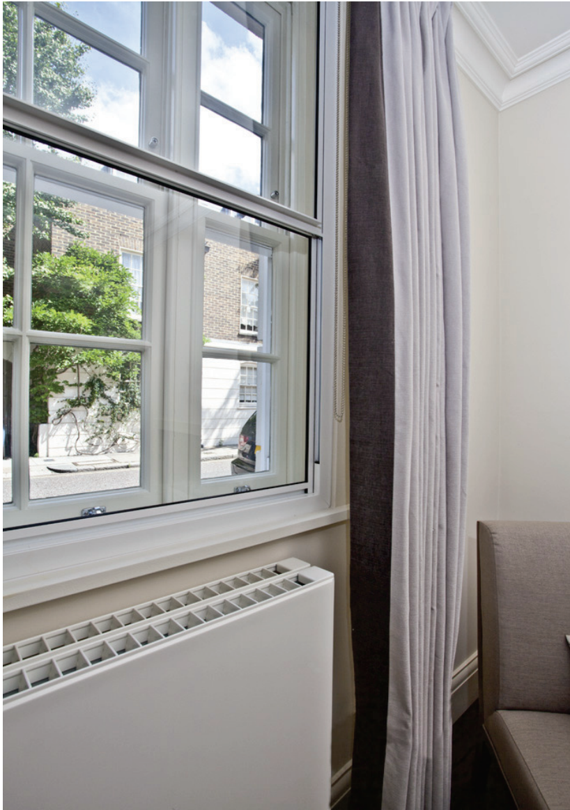
Secondary glazing at 15 Passmore Street, Grosvenor Plc
