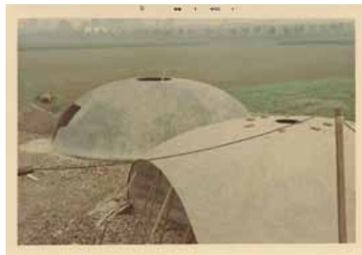
Binishell construction, Castelfranco, Italy 1966, Photograph Dante Bini: Building With Air .
