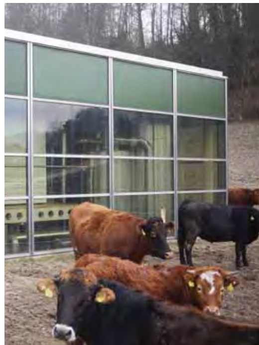
Swiss Federal Railways (SBB) training centre at Löwenberg, Switzerland (1978-1982) by architect Fritz Haller. Part of ongoing study into systems building. Photograph W. McLean, 2012.
