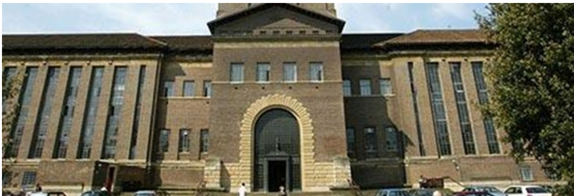
Cambridge University Library, another pilot project. Source: www.cambridgeretrofit.com .
