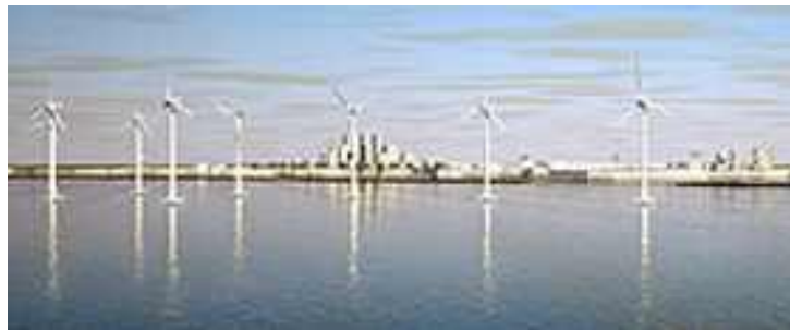
Wind farm at Caofeidian International Eco-City. Courtesy of SWECO.
